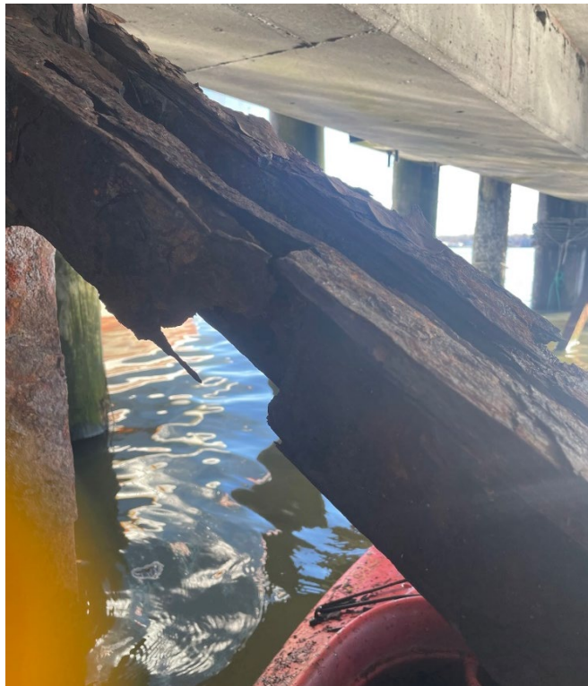
Picture #17 Typical Diagonal Bracing Corrosion (Poor)
