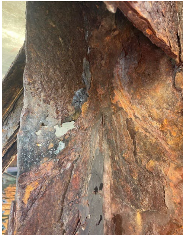
Picture #18 H-pile Corrosion in Service Pier 1.
